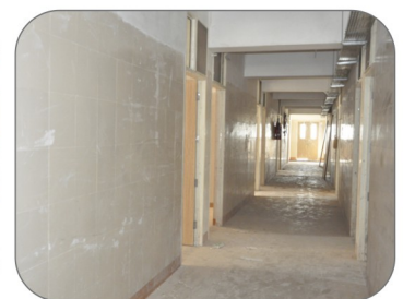
New PG accommodation
