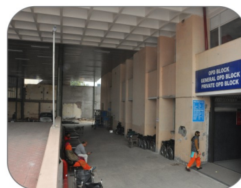
Shed Near OPD Block
